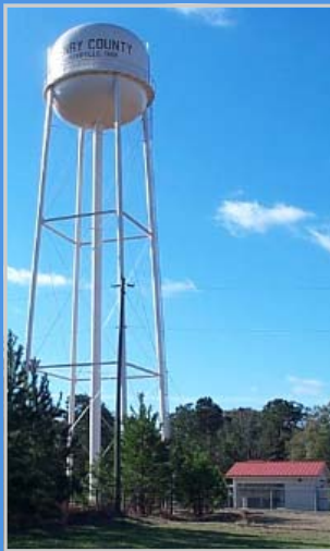
Above: 150,000 Gallon Elevated Water Storage Tank and 400 GPM Well in Shorterville Constructed in Phase 7
